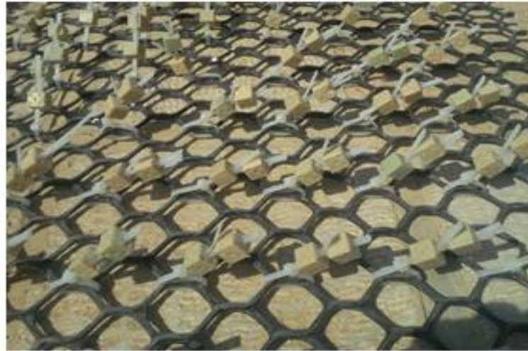
Fig-3. The method of placing the anchor on the geome
