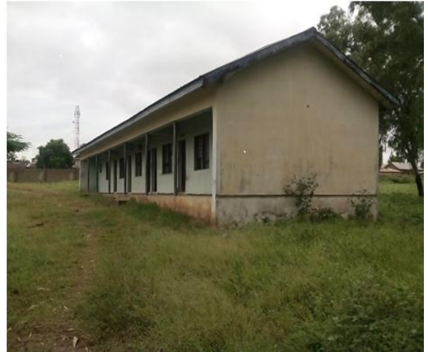
Fig-2. Divisional Office of Forestry Department in Jalingo Source: Fieldwork 2016
