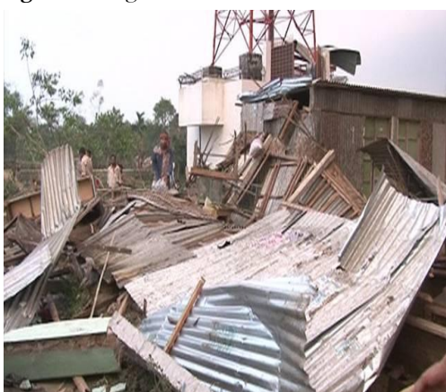
Fig-5. Damaged structures and houses
