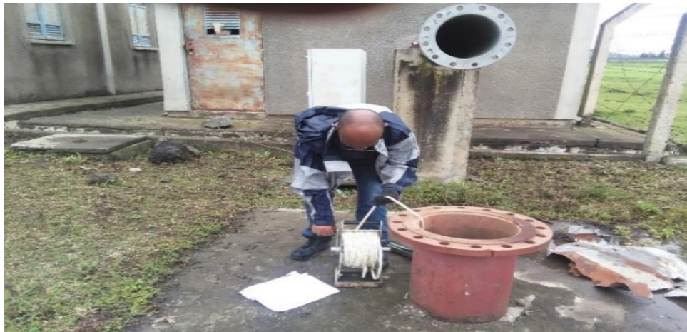
Figure-4. One of the dismantled wells due to groundwater level decline.
