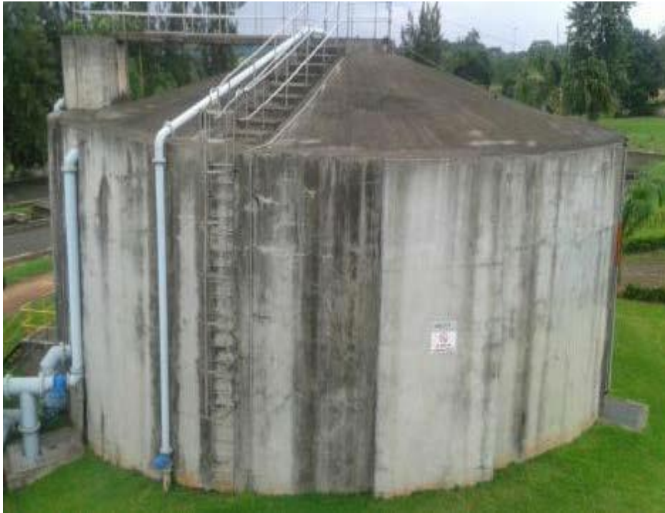
Fig-5. The 3000 m 3 digester at Tzaneen WWTW
