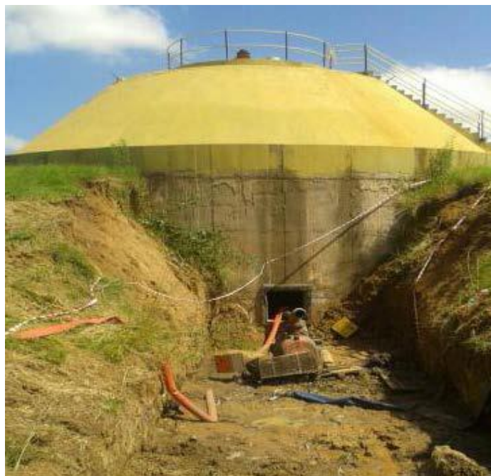
Fig-4. Anaerobic digesters being de-sludged. Source: SALGA (2015)
