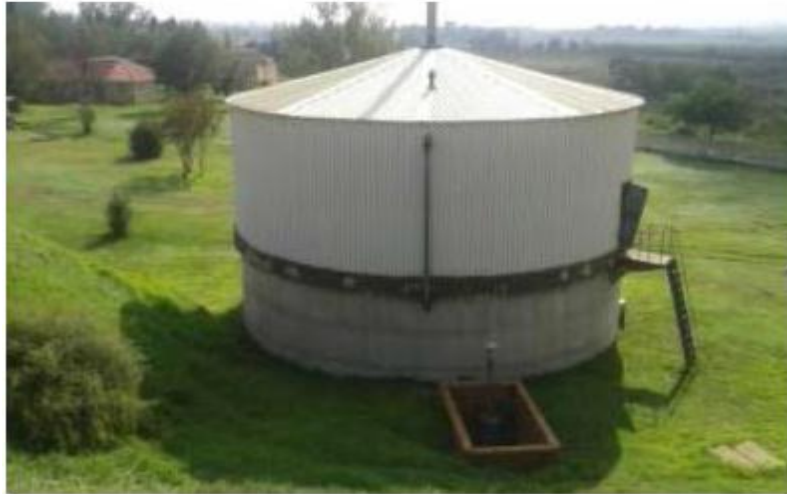
Fig-3. 1000 m 3 biogas digester for human excreta Source: South Africa Local Government Association (SALGA) (2015)
