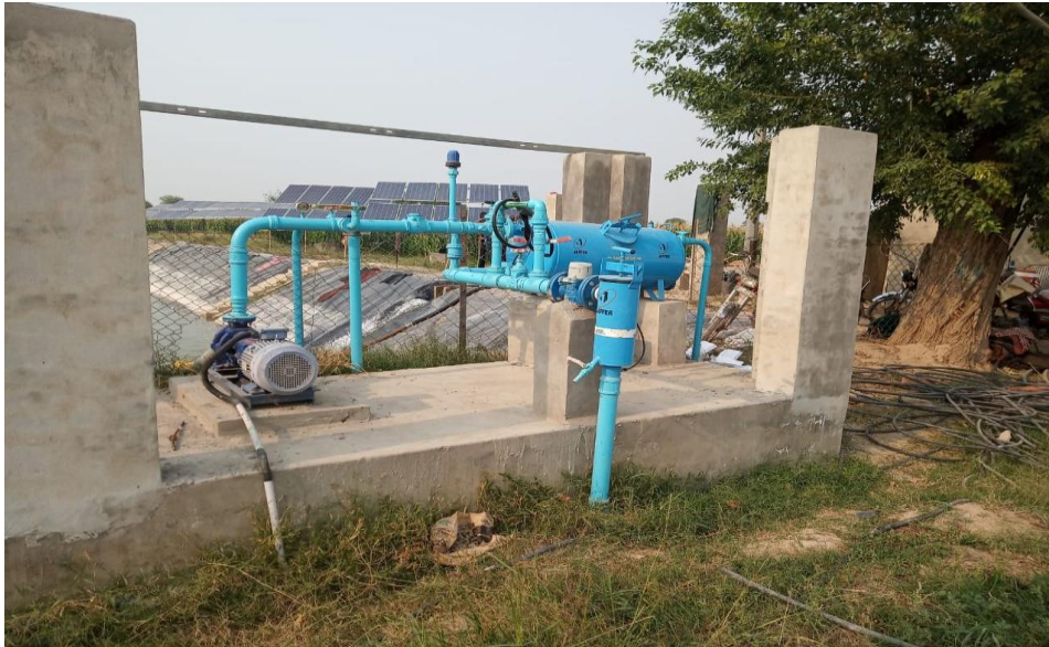
Figure-1. Drip System Head Unit.
