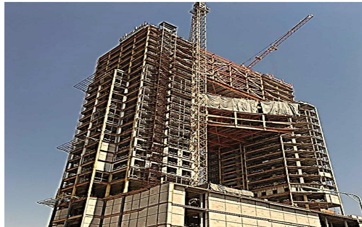
Figure-3. South facade of YAS Tower
