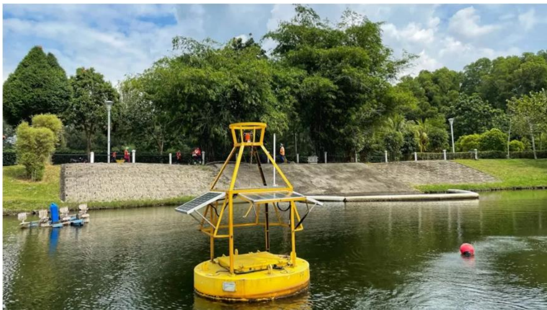
Figure 5. Putrajaya corporation supervisory control and data acquisition (PJC SCADA) Line lake water quality monitoring system at Putrajaya Lake (Photos was taken by Nur'ain Azhar).
