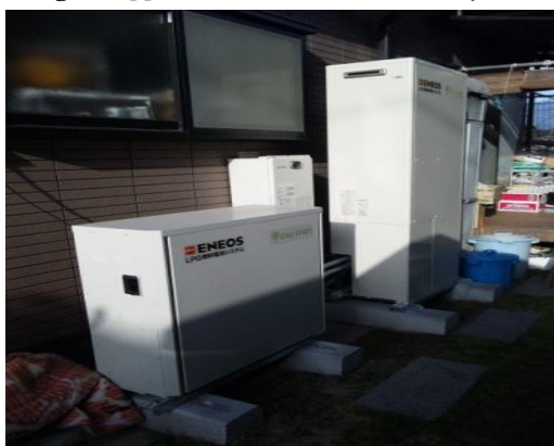
Fig-1. Appearance of a 1 kW PEFC system
