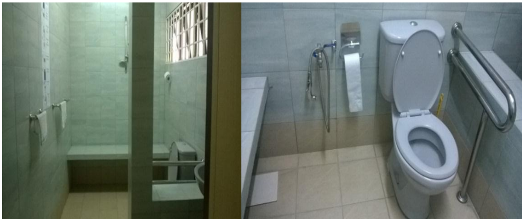
Figure-5. Accessible toilet that is purposefully built to meet the needs of the disabled people in case study 2, Petaling Jaya daycare centre
