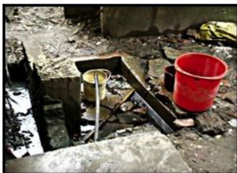
Figure-3. Water Pipeline
