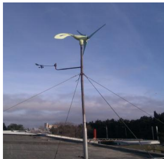
Figure-8. The general view of wind energy plant
