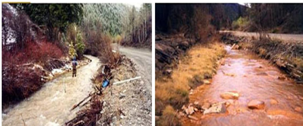
Plate-2. Destruction caused by erosion in Ayoguri and Afowa
