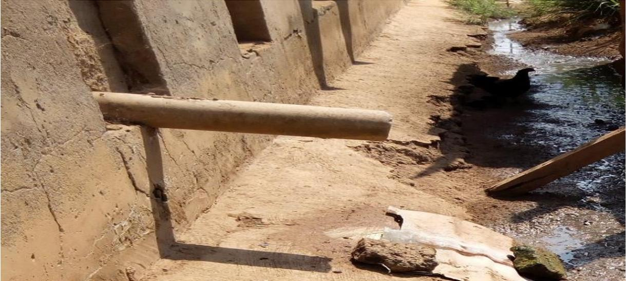
**Figure 2.** Waste water from bathroom contributing to in-street wastewater in Ilesa, Osun State.
