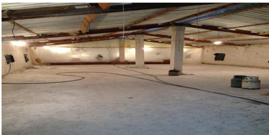
Figure-2. Livestock buildings.
